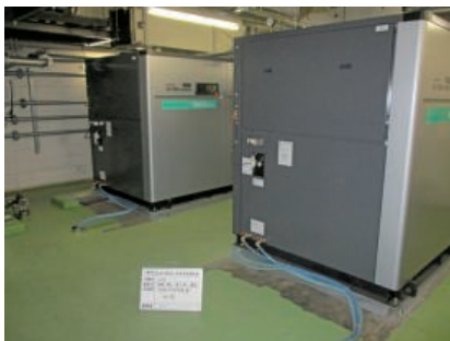
Compressor after replacement (the new type consumes 30% less energy)
