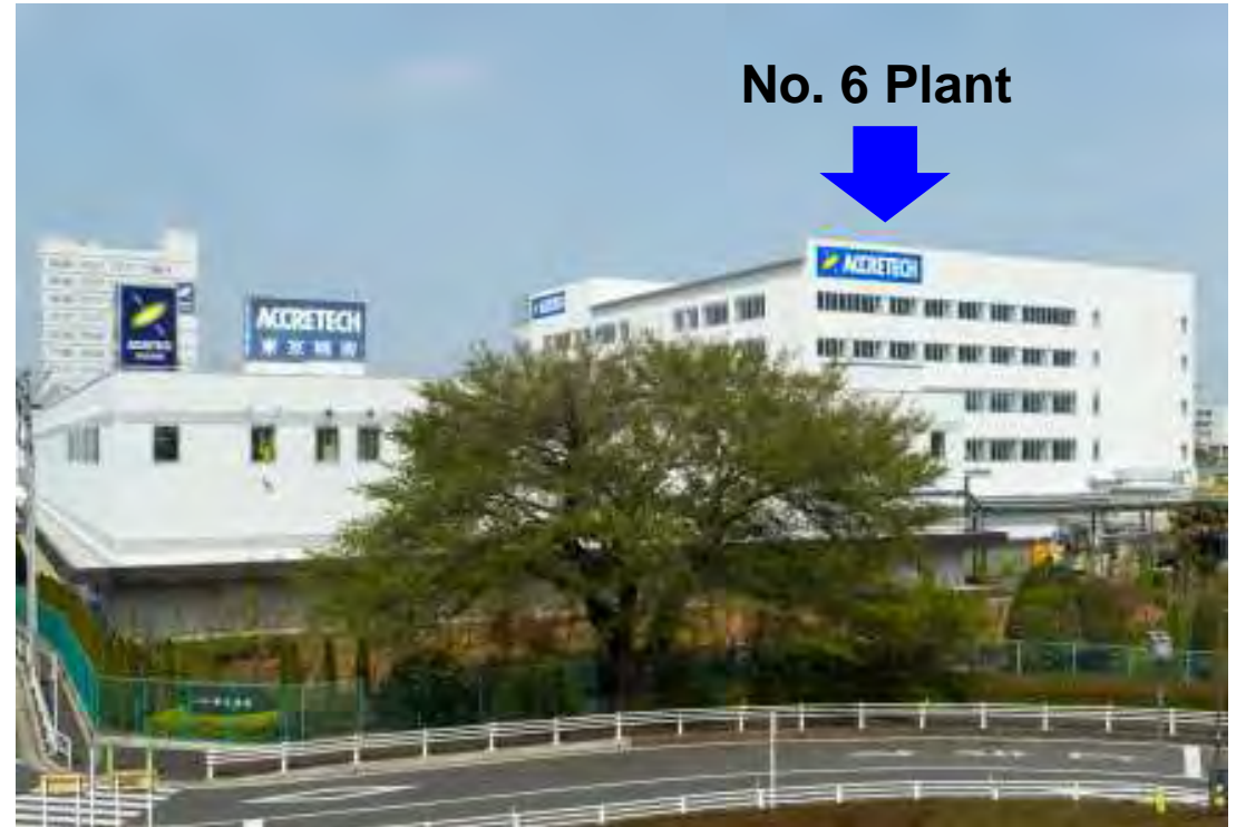
Hachioji No.6 Plant (Tokyo, Japan) Construction completed in May 2016
