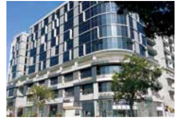
Accretech (Singapore) Pte. Ltd.
